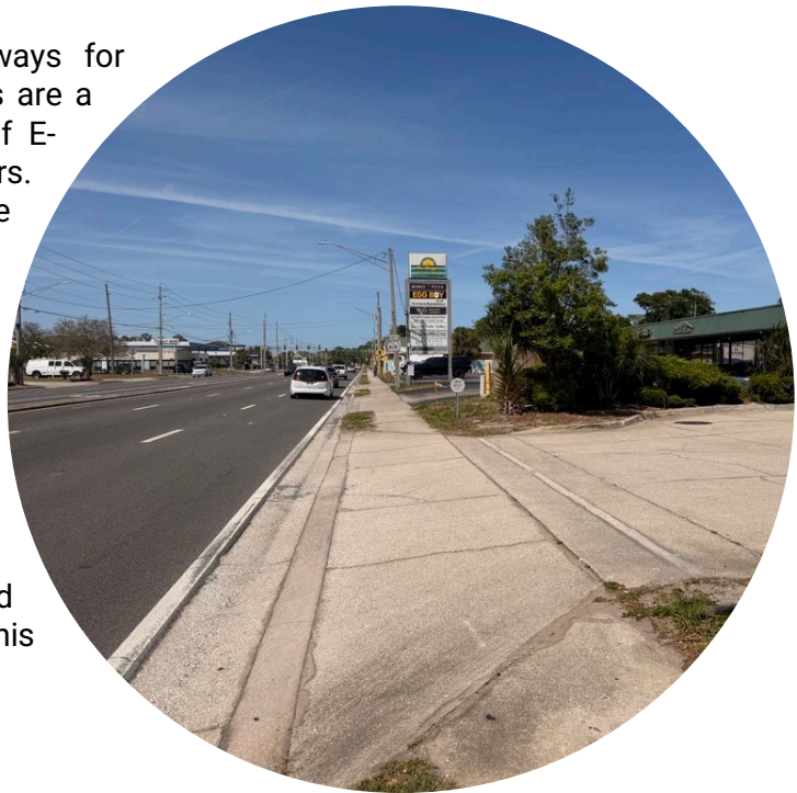
Photo 4. Driveways on Mayport Road (A1A) Facing North
