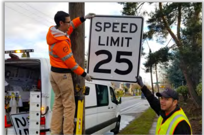
Workers replacing speed limit signs in Portland, OR.
