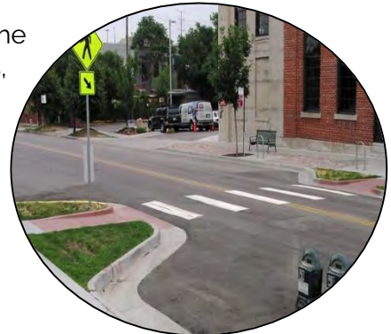
Curb extension example. Image Credit: Richard Drdul
