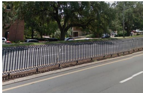
Steel Loop Fence
